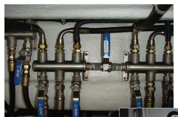
Left, steering manifold with bypass valve labeled. Below, a steering oil reservoir equipped with an air pressure gauge and oil level windows.
