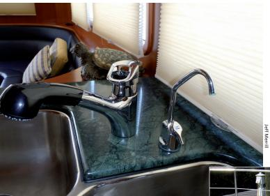
Seagull IV water purifier. This is a separate freshwater tap that has a special filter and provides clean drinking water for making coffee, tea or for use in cooking — soups, etc.
