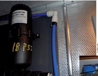
Above, a freshwater accumulator tank with the pressure marked. Right, a freshwater tank inspection top that has been properly labeled to ease troubleshooting.
