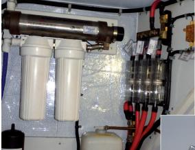
Above, this water fixer unit has a UV sterilizer and dual-filter cartridges. Right, hose bib caps close off the ends of these fixtures and prevent leaks. pump is not designed for prolonged use and, if you run a lot of water through it be aware that the pump motor can overheat and stop. I like to see a light diode on the electrical panel that illuminates when the pump runs; if
