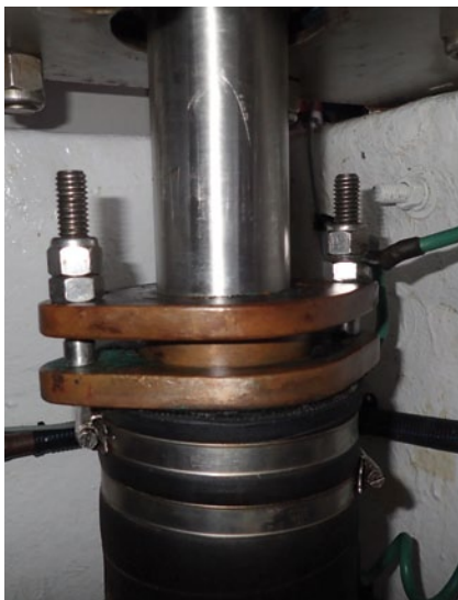
A typical rudderpost, an often overlooked area for producing leaks.
